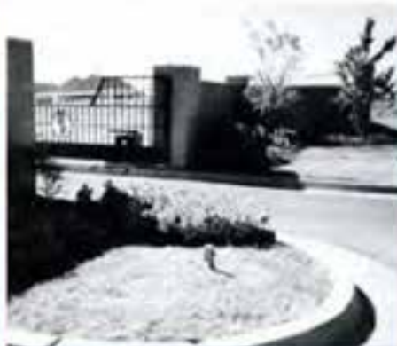
Braden Park Development
