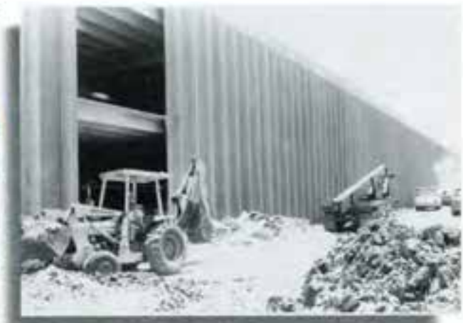
Kirkpatrick Center under construction
